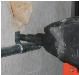
12HSMPO34 clip assembly used to secure conduit
