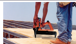
Plywood attachment—using TrakFast plywood to steel pin
